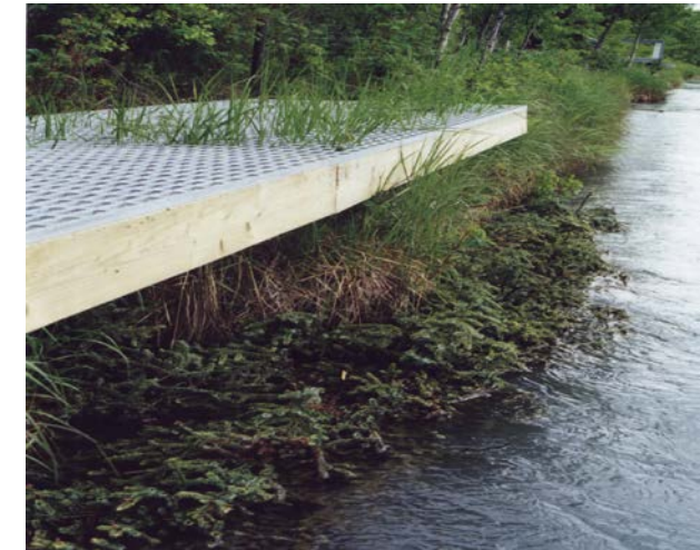
An example of a light penetrating grate walk above a restored riverbank. This project is eligible for a tax credit and partial cost reimbursement.
