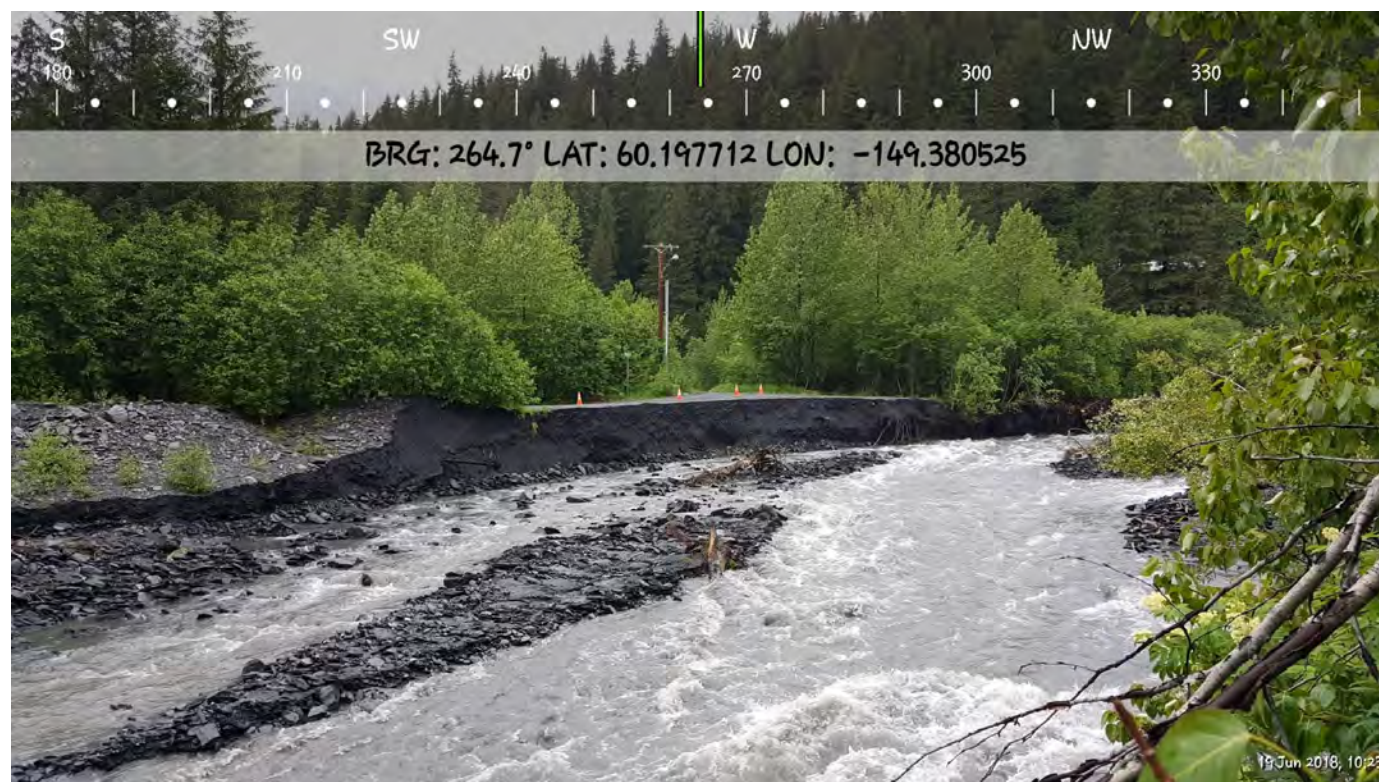
Looking across Lost Creek to the eroded Tongass Ln cul-de-sac.
