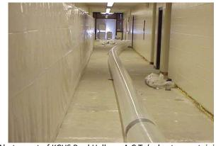
Abatement of KCHS Pool Hallway A.C.T. (asbestos containing tile) and mastic.
